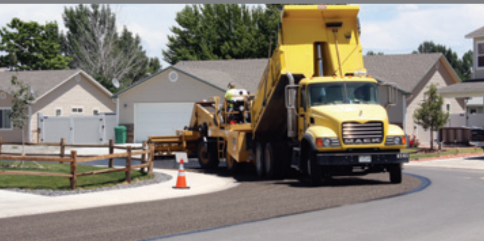
Above left: With Grand Mesa, world's largest flat-top mountain in background, HYPAC rollers compact chip seal application in a residential area.
